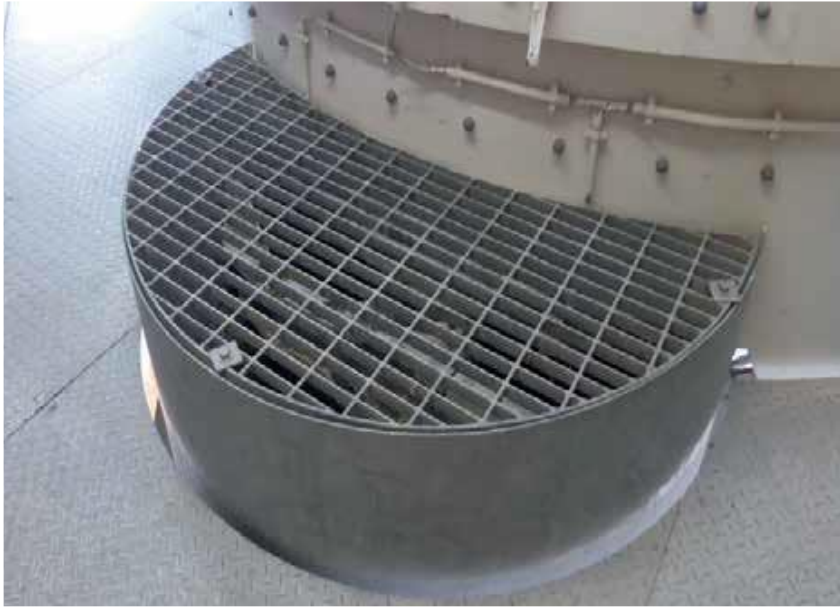
Picture 32: Example of mixer discharge point and inspection hatch guarding
