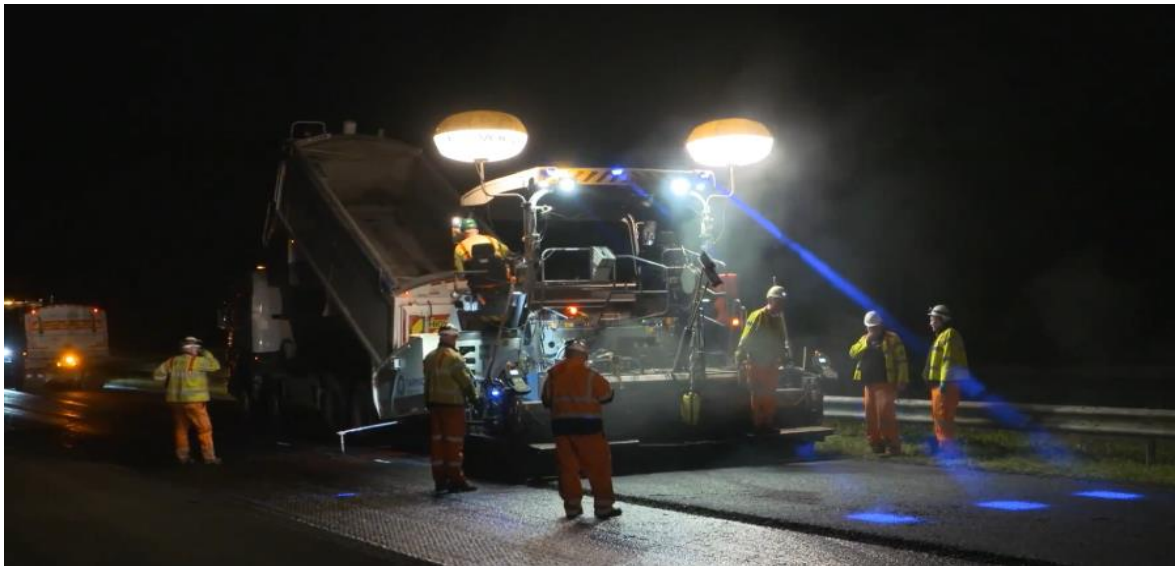
Video 40: Example of danger zone light system - 5+2 blue lights (Tarmac)
