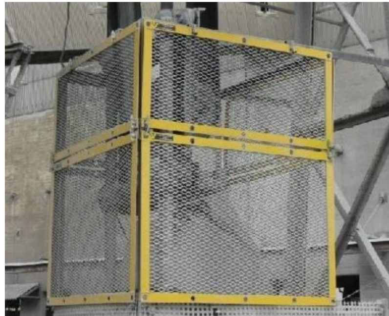
Picture 3: Example if gravity take up unit guarding
