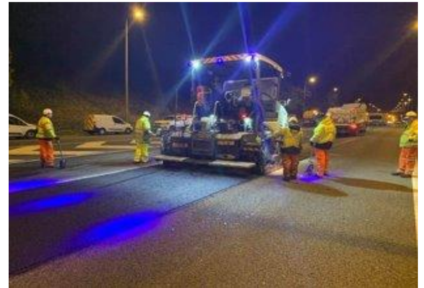
Video 39: Example of danger zone light system - 5+2 blue lights (Tarmac)
