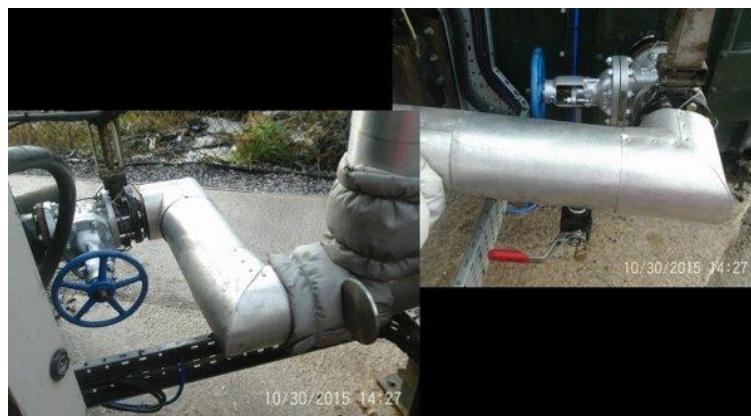
Picture 46: Example of Block and Bleed Valves
