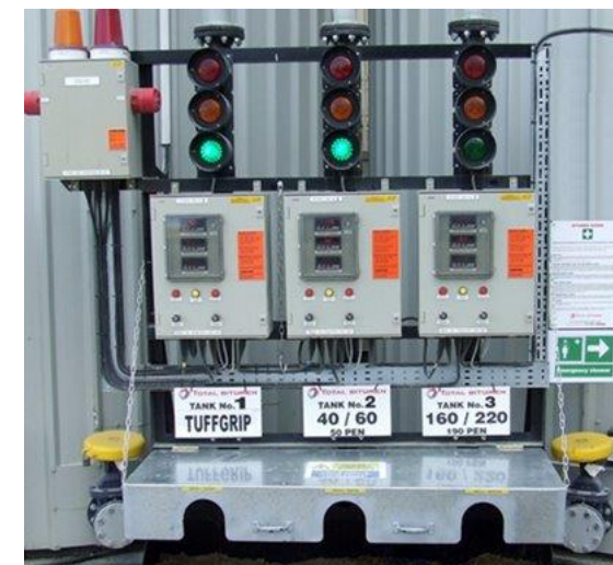
Picture 47: Example of High Level Alarm (HLA) / High High Level Alarm (HHLA)
