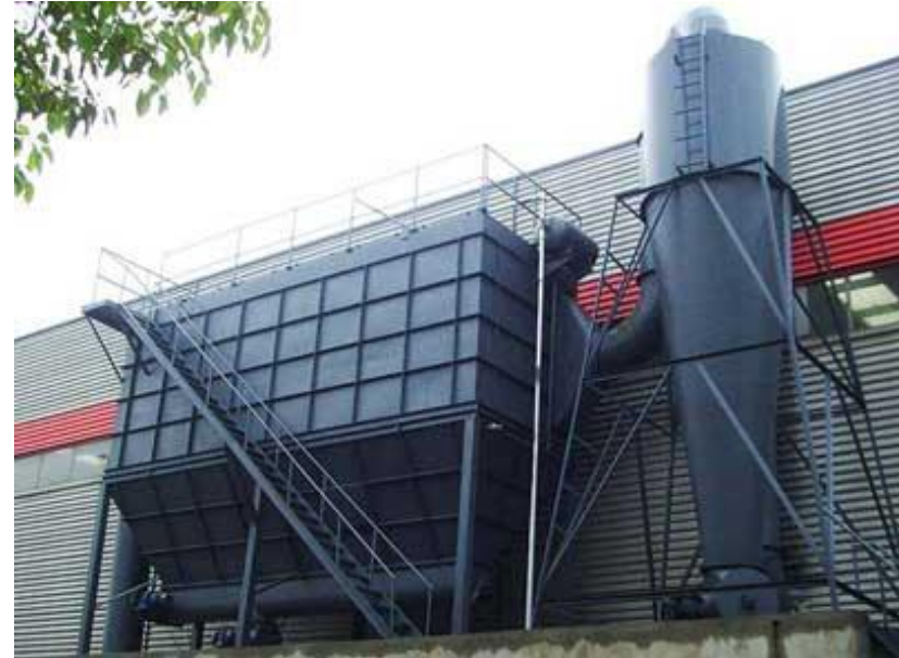
Picture 16: Examples of bag filter units with safe access and working platforms
