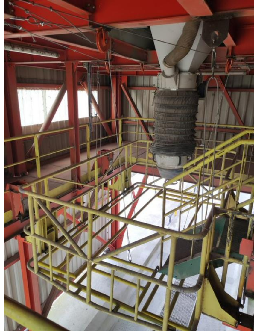
Picture 38: Examples of railing to provide fall protection while opening / closing tanker hatches
