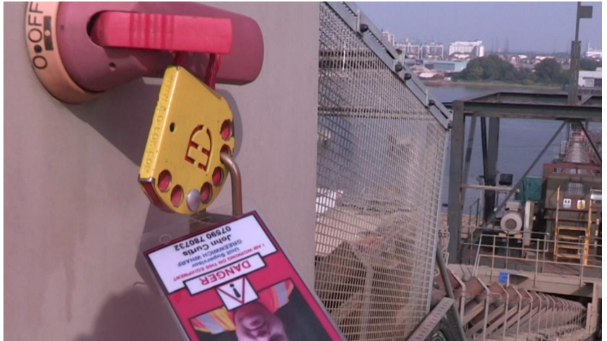
Picture 8: Examples of isolators located close to the machine
