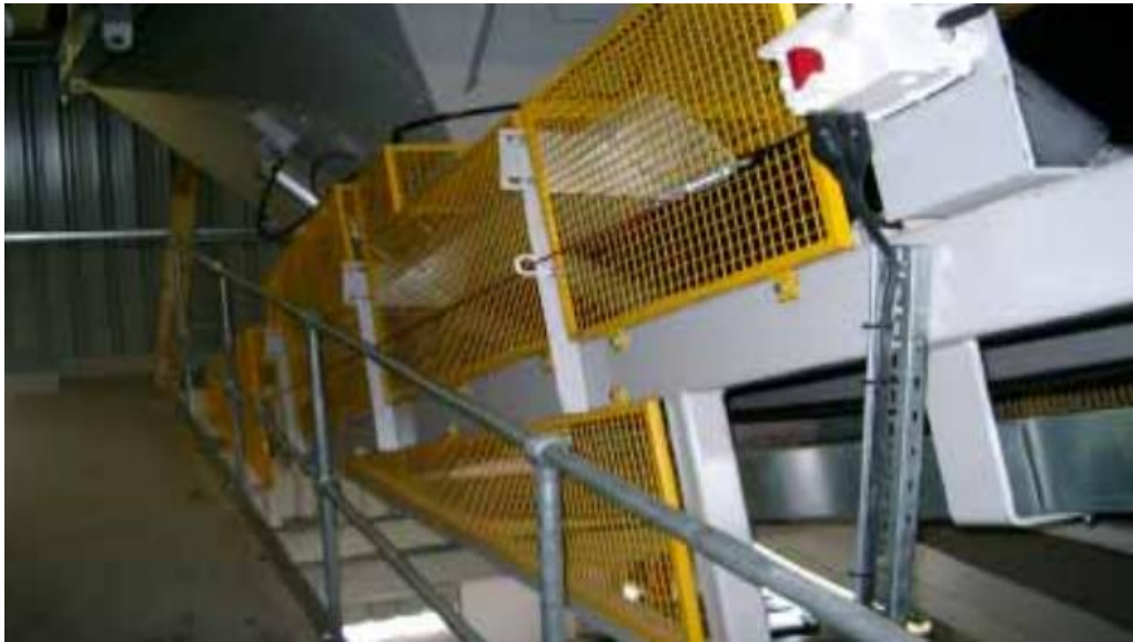
Picture 6: Example of skirting guard
