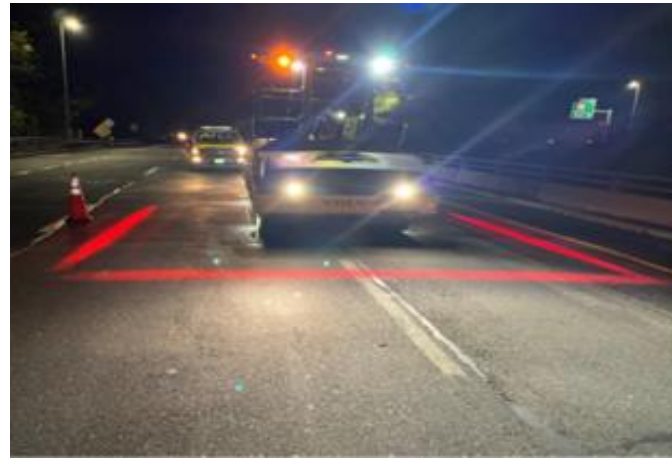
Picture 71: Example of danger zone light system - Red lights
