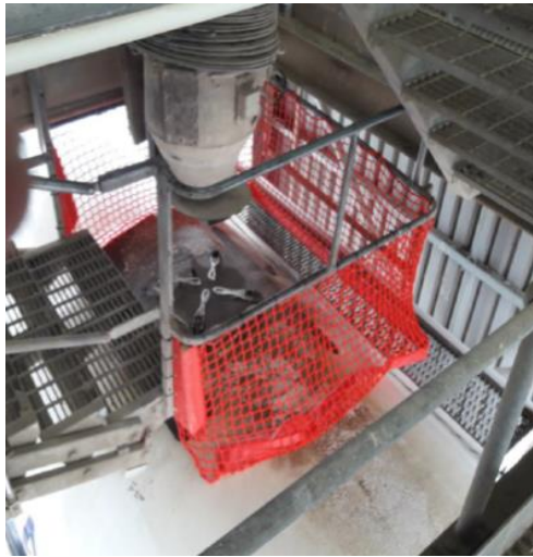
Picture 38: Examples of railing to provide fall protection while opening / closing tanker hatches
