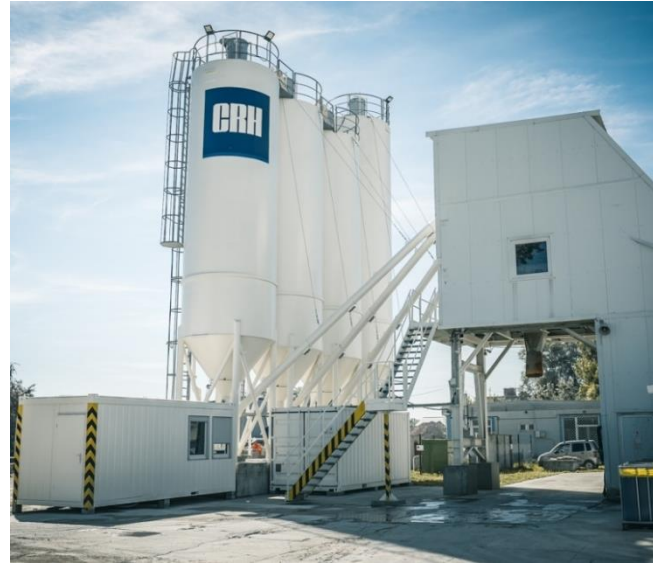
Picture 18: Examples of access ladder: rising more than 3.5 m should be fitted with hoops commencing at 2.5 m from ground level. The hoops should be spaced at 1.2 m intervals and the internal clearance of the hoops should be in the region of 0.8 m. For high rise ladder access, there must be a rest platform every 6 m on the access ladder.
