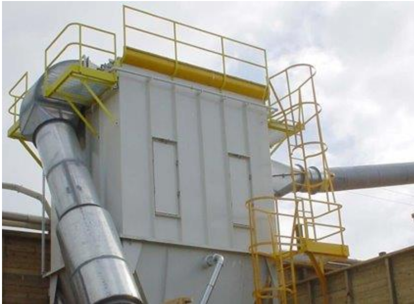
Picture 16: Examples of bag filter units with safe access and working platforms
