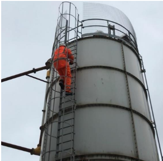
Picture 18: Examples of access ladder: rising more than 3.5 m should be fitted with hoops commencing at 2.5 m from ground level. The hoops should be spaced at 1.2 m intervals and the internal clearance of the hoops should be in the region of 0.8 m. For high rise ladder access, there must be a rest platform every 6 m on the access ladder.
