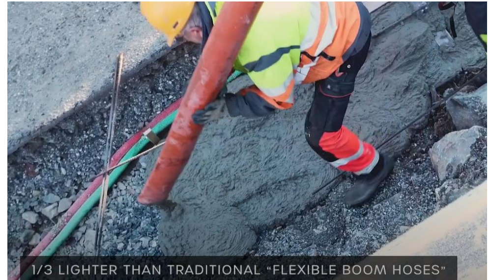
Video 68: Example of Lightweight and Flexible Boom End Hose (Mandals)
