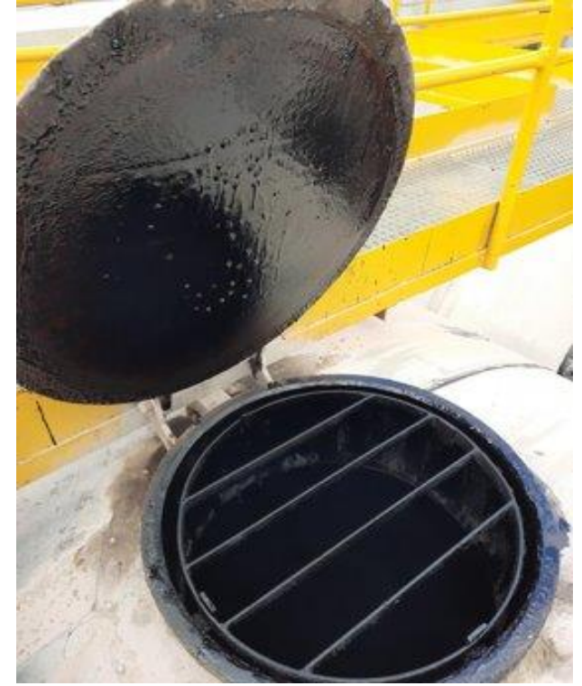
Picture 42: Example of manhole fitted with grid
