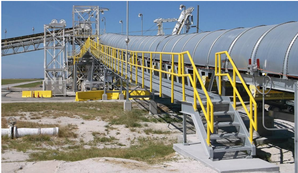
Picture 13: Examples of catwalks along the belt and safe working platforms for head drum maintenance
